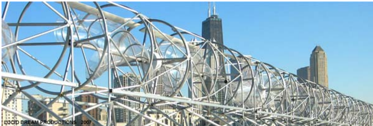
Fig. 5 - Horizontal Aerotecture wind turbine.
